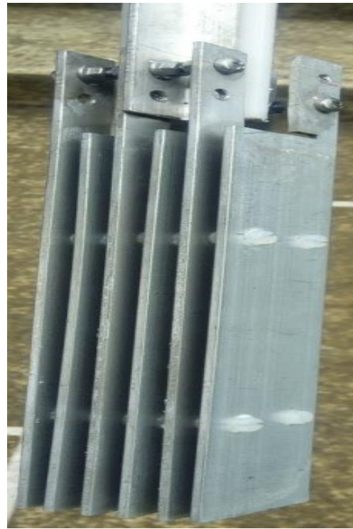
Figure 7: Power supply in a parallel monopolar connection
